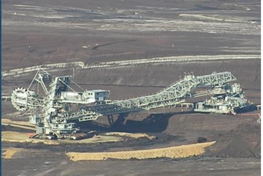
An operational Bucket Wheel Reclaimer transferring coal onto an overland conveyor.
